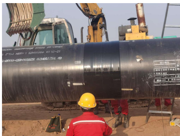
Induction heating application
